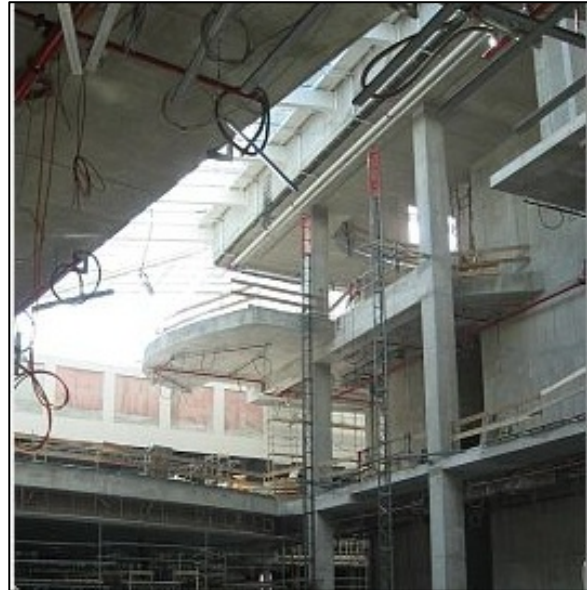
Figure 8: A concrete structure and electrical wiring typical of German construction.
