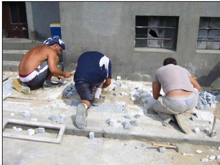
Figure 11: Three gypsy construction workers placing a brick sidewalk in the traditional Czech style.
