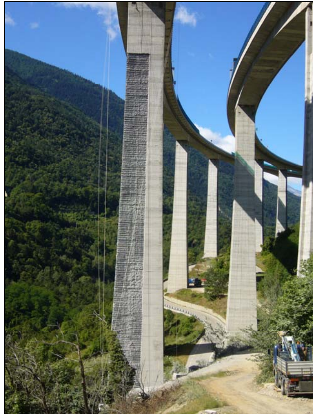
Figure 10: Repair of the Ramat Bridge near Turin, Italy. The concrete surface is removed, and a new surface is applied with additional reinforcement.
