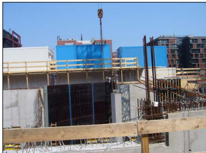
Figure 6: An apartment utilizing the combination of pre-cast and cast-in-place concrete construction in
