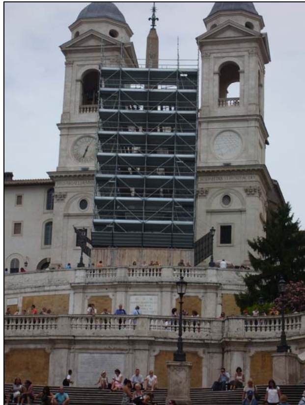
Figure 3: Renovations and repairs near the Spanish Steps in Rome, Italy.
