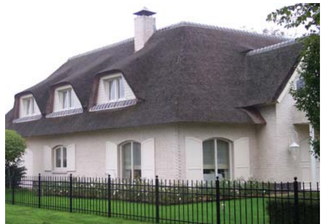
Thatched roof house in Etten-Leur
