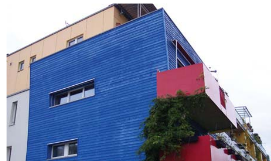
ISIS Passivehaus in Vauban
