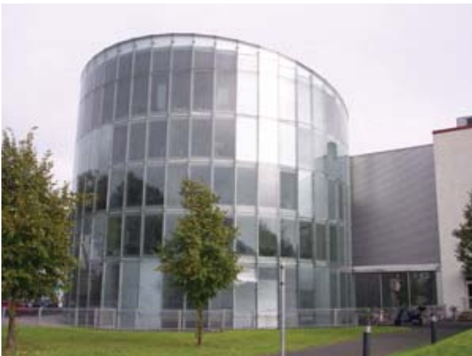
Norman Foster Office Building, Duisburg
