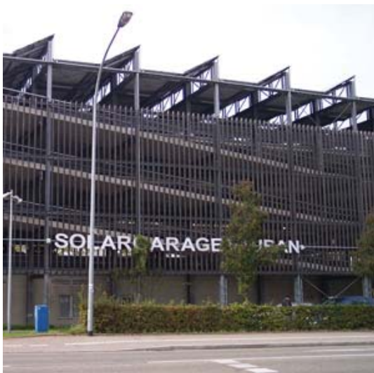
Solargarage: Rooftop PV panels generate electricity for the grid in this Vauban neighborhood parking structure.
