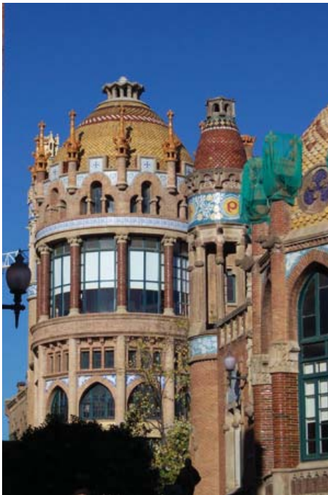
Another building at the hospital
