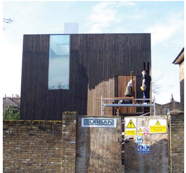
Ed Reeve's house being constructed
