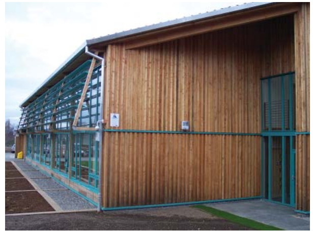
Natural, unfinished wood is the main building material in the Scottish Forestry Commission's new building
